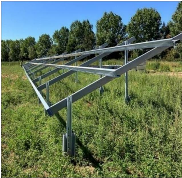
Plate 3.14: Example construction piling for the installation of the Solar PV mounting structures
