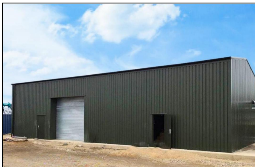
Plate 3.11: Example of a Collector Compound
